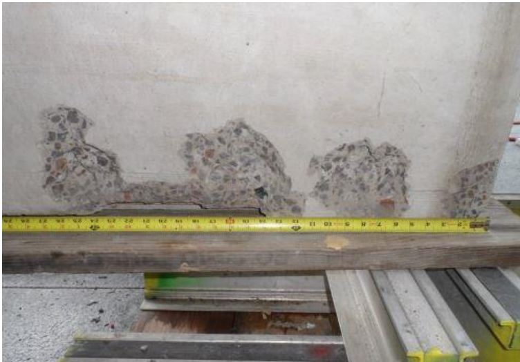
Concrete panel intentionally chipped for anchorage installation
