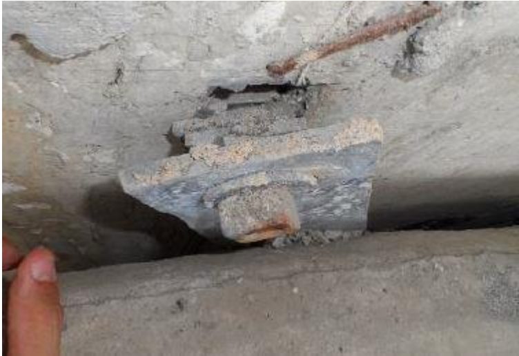
Strap anchor. Shims filling gap, strap bent
