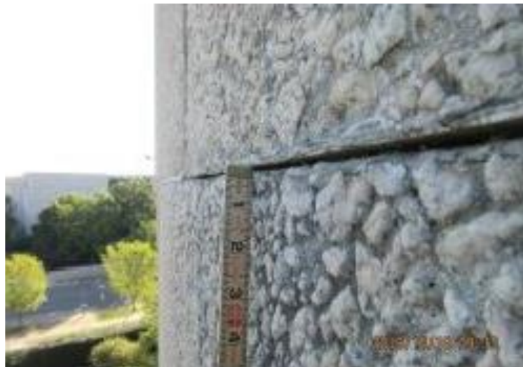
Uneven spacing between panels
