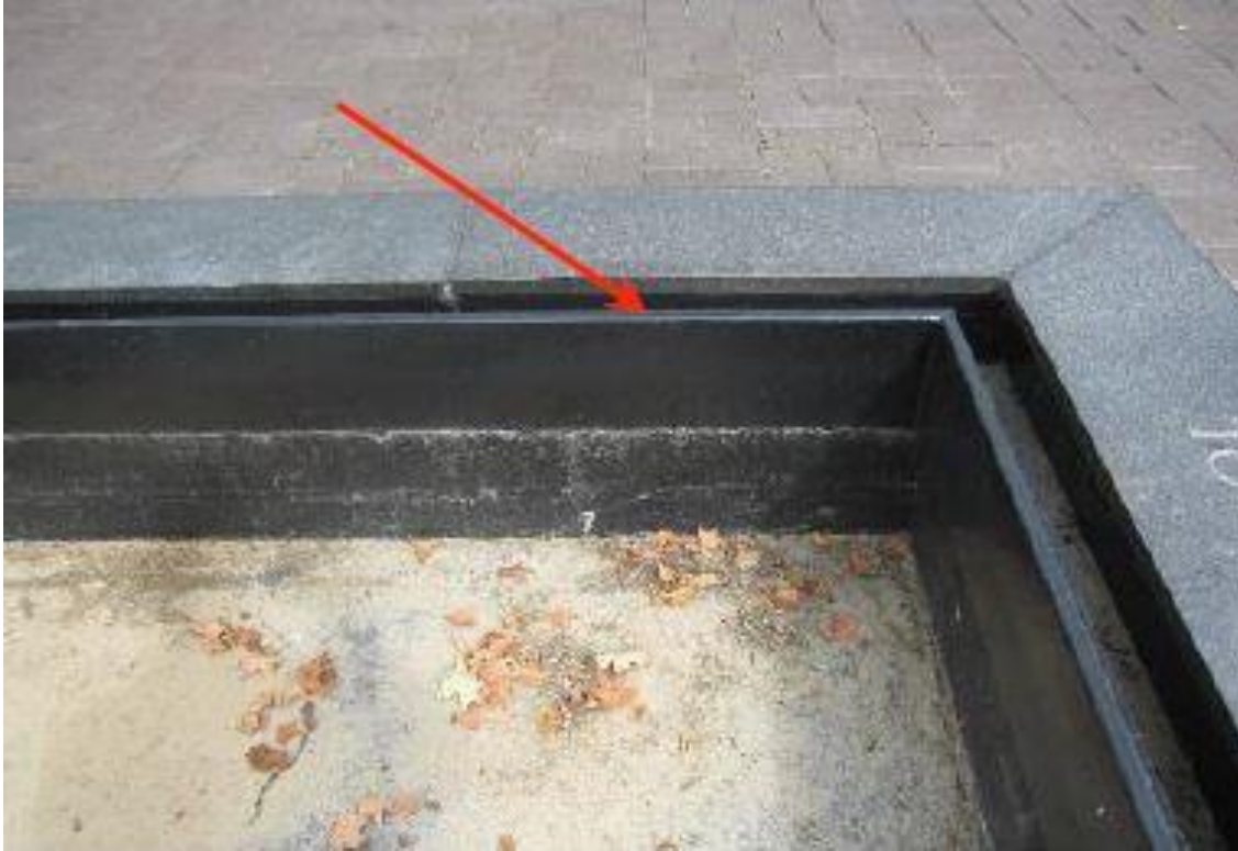
Pool perimeter condition, metal fin separates pool from perimeter gutter
