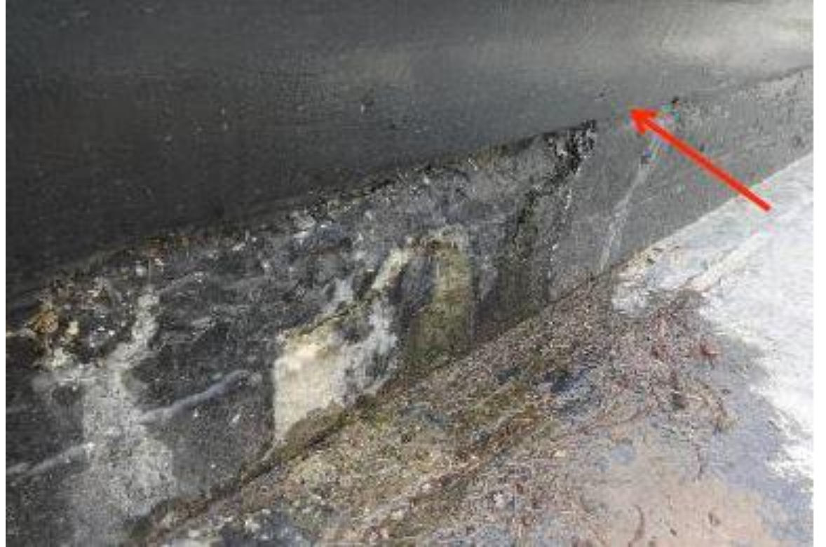
Pool perimeter, deterioration of concrete and waterproofing
