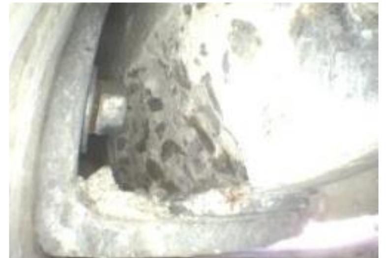
Concrete spalling adjacent to relieving angle bearing surface
