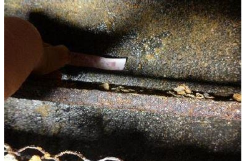
Concrete back-up wall, Water saturation
