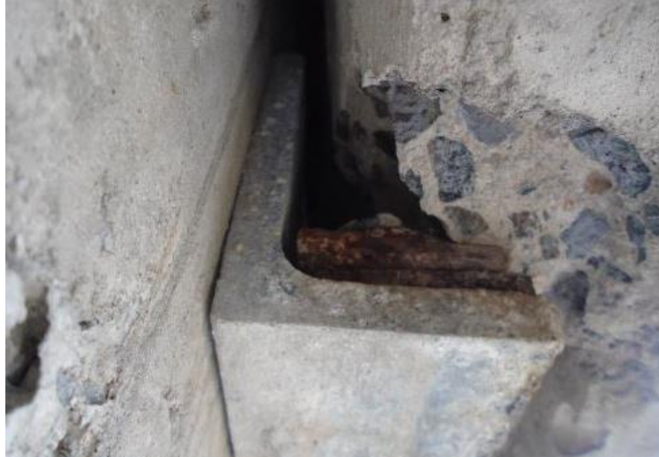
Relieving angle. Corrosion, spalling, and uneven panel bearing
