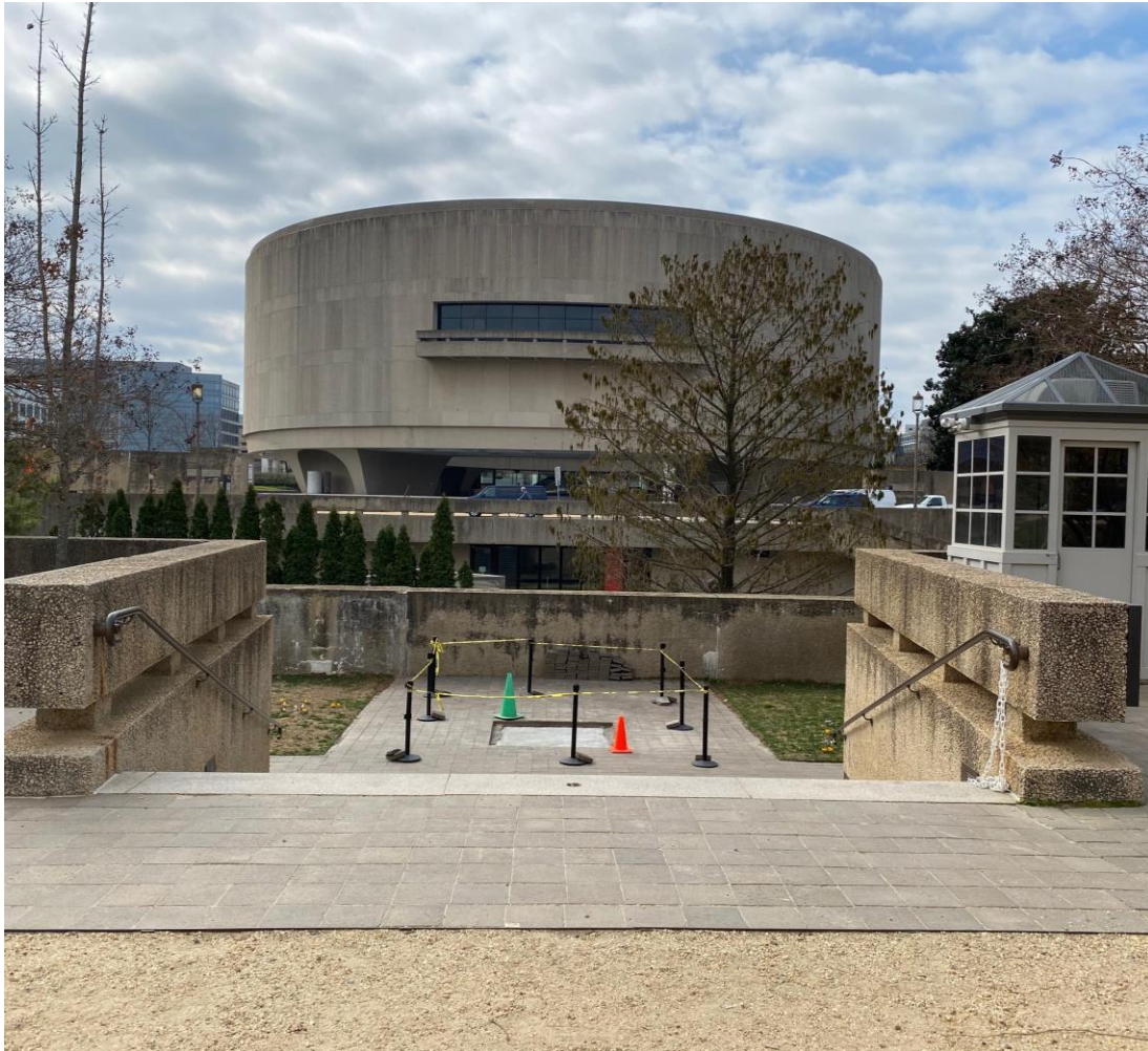
Existing North Stair
