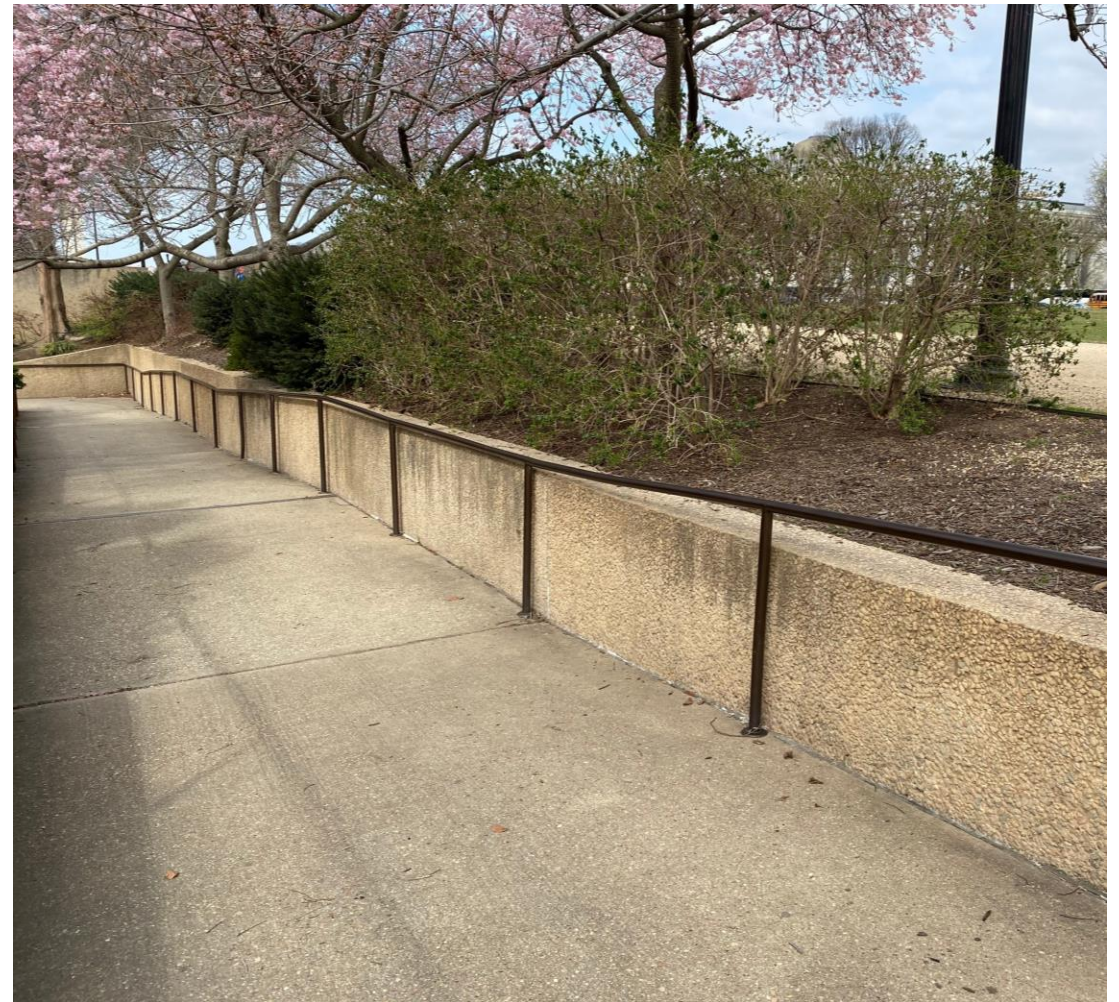
Existing West Ramp
