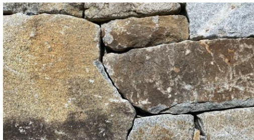
3 - Stacked Stone Walls
