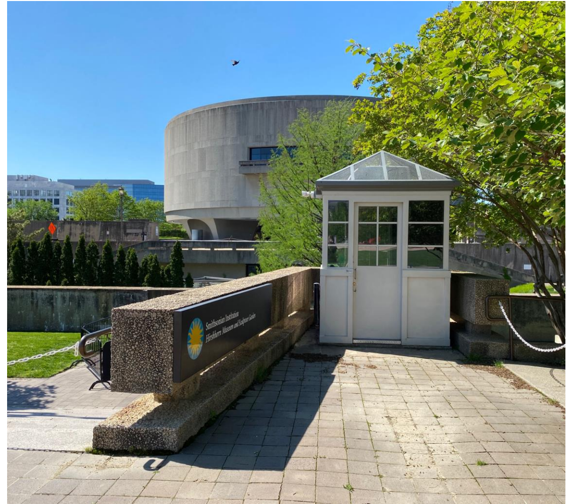
Existing Guard Booth on 8 th Street Axis
