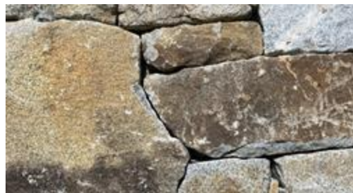
3 - Stacked Stone Walls
