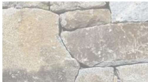
3 - Stacked Stone Walls
