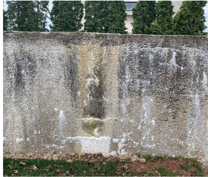
1974 Wall, Alkali Silica Reaction
