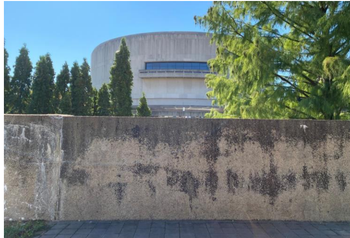
Inner Partition Wall - Alkali-silica Reaction
